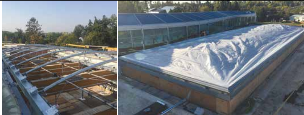
Far right: ETFE skylight above panda exhibit being inflated with a blower.
