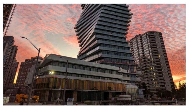
PHOTO COURTESY ELLISDON - Upon completion, M City in Mississauga, Ont. will be an eight-tower, 15-acre, 4.3-million-square-foot development. For the M1 and M2 twisting towers, walking columns were installed for easier rebar placement and more straightforward formwork.
