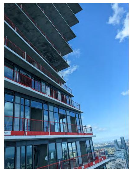
COURTESY ELLISDON - Approximately 53,000 cubic metres of concrete was placed in M1, whereas the volume in M2 is closer to 56,000 cubic metres.
