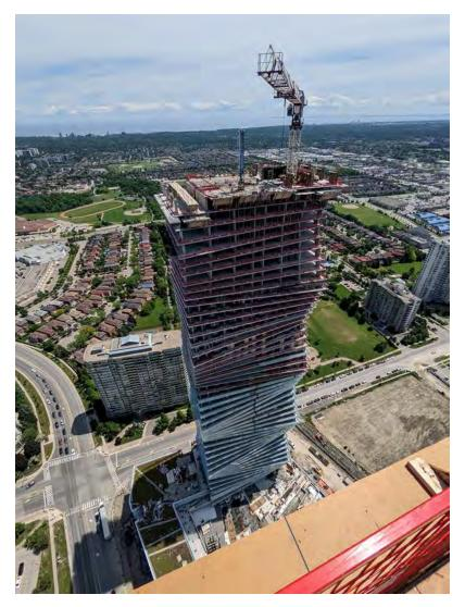
PHOTO COURTESY ELLISDON – A conventional fly form system was used in the construction and the concrete was pumped to each floor, a process that did require some planning and set up time.
