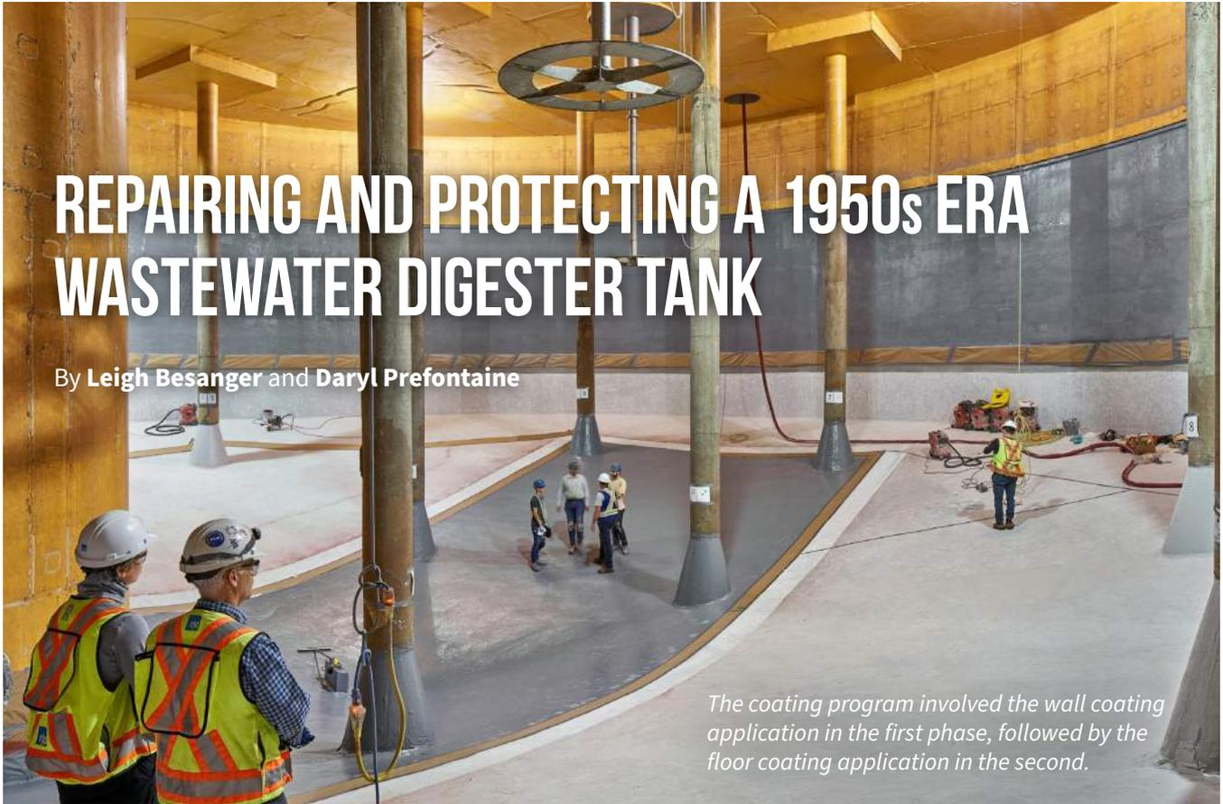
*The coating program involved the wall coating application in the first phase, followed by the floor coating application in the second.*
