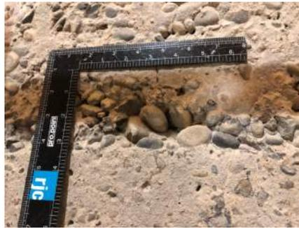
*Poorly consolidated and non-encapsulated aggregate.*
