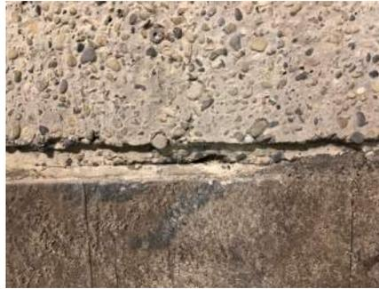
*Voids and debris at pour-joint (bare concrete above joint, existing coal tar coating below).*
