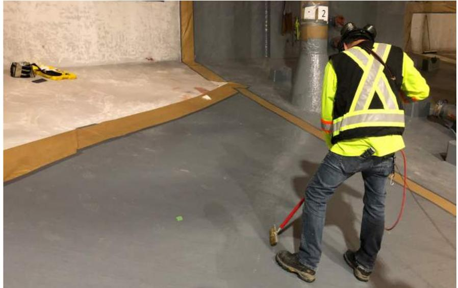
After each round of holiday/spark testing, pin-hole and coating discontinuity repairs were performed and retested.
