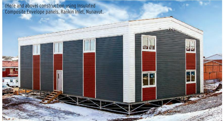
and turn on the heat. Due to the nature of our ICE Panels with their built-in insulation and vapour barrier, once the building is erected and windows and doors are installed, the heat can be turned on and construction can continue.
