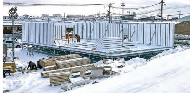
(Here and above) construction using Insulated Composite Envelope panels, Rankin Inlet, Nunavut.
