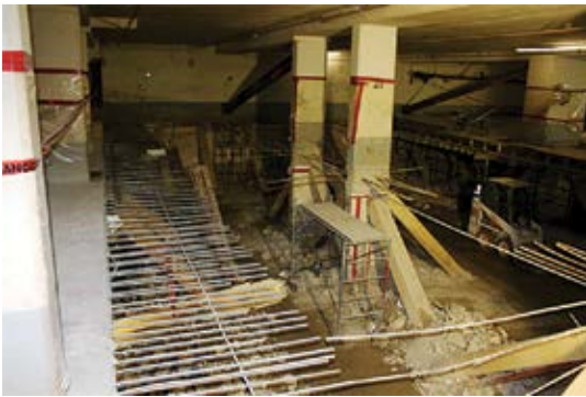
Fig. 7: Slab removal and replacement operations were carefully sequenced over several phases to maintain lateral support for the building walls and columns, while minimizing bracing and shoring requirements
