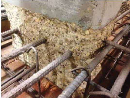
Fig. 8: Existing slab and slab-band reinforcing steel were maintained, abrasive-blast cleaned, and reincorporated into the new work at the perimeter walls, core walls, and interior columns
