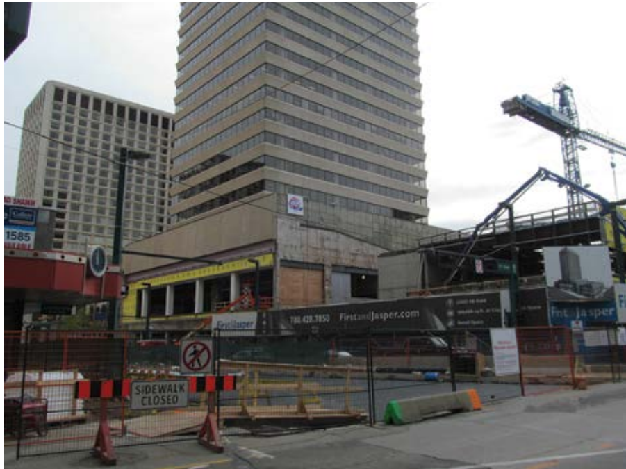
Fig. 1: Overall view of project site during construction
