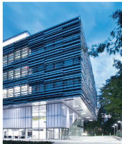
Langara College Science & Technology Building | LEED® Registered
