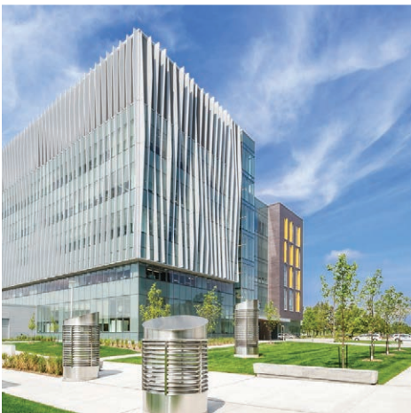
University of Toronto Scarborough | Environmental Science and Chemistry Building | LEED® Gold
